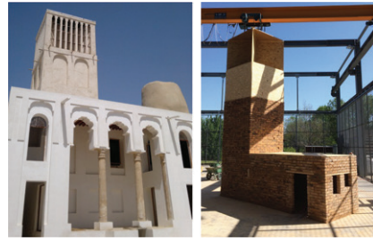
Figure 6. Original Badgir (left) and the half-scale Badgir (right).
